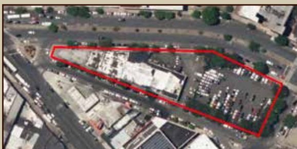
$23.6M 1st - Development Site Bronx, NY
