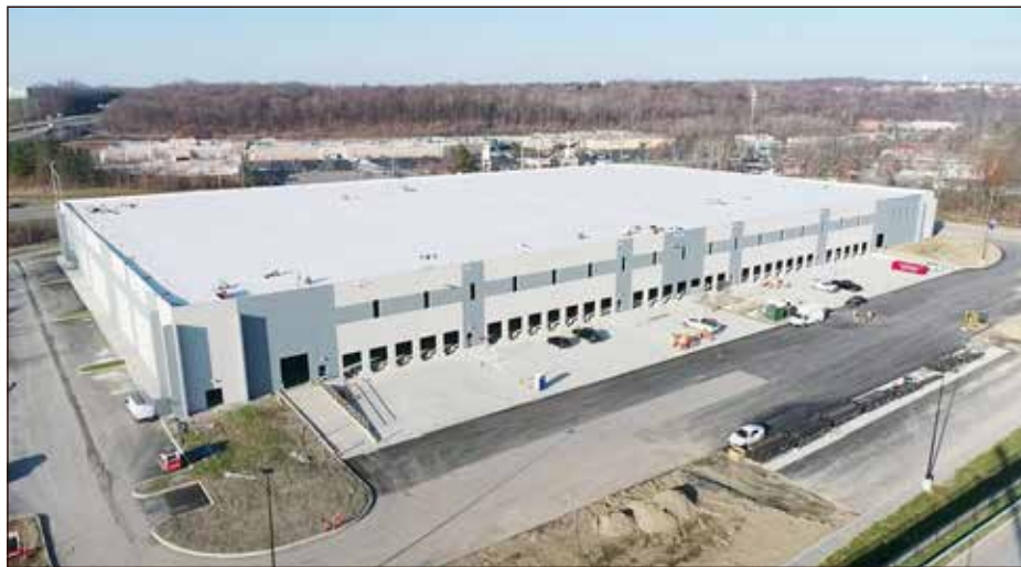
Tesla will occupy 1396 Route 300 in Newburgh and utilize the property as a distribution facility.
