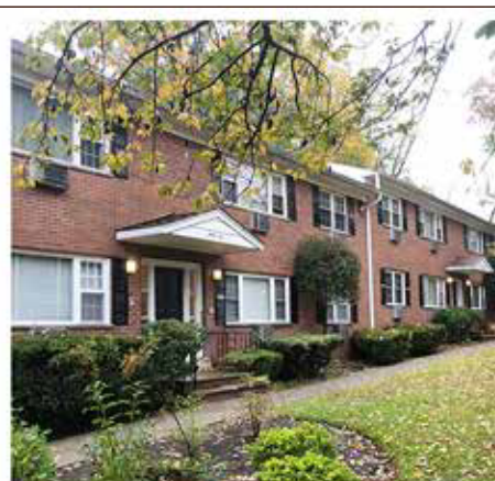
Henry Street Apartments Pearl River, NY
