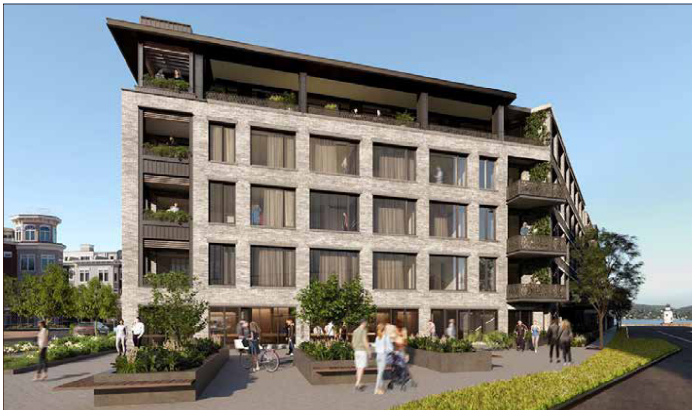
The financing will be used to develop The Daymark, a 100-unit waterfront condominium at the Edge-on-Hudson in Tarrytown.
