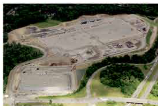
1MM+ SF SPEC BUILDINGS (2) 1396 Route 300 Town of Newburgh
