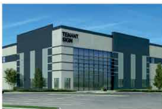
80,000 SF SPEC BUILDING 18 Leonards Drive Town of Montgomery
