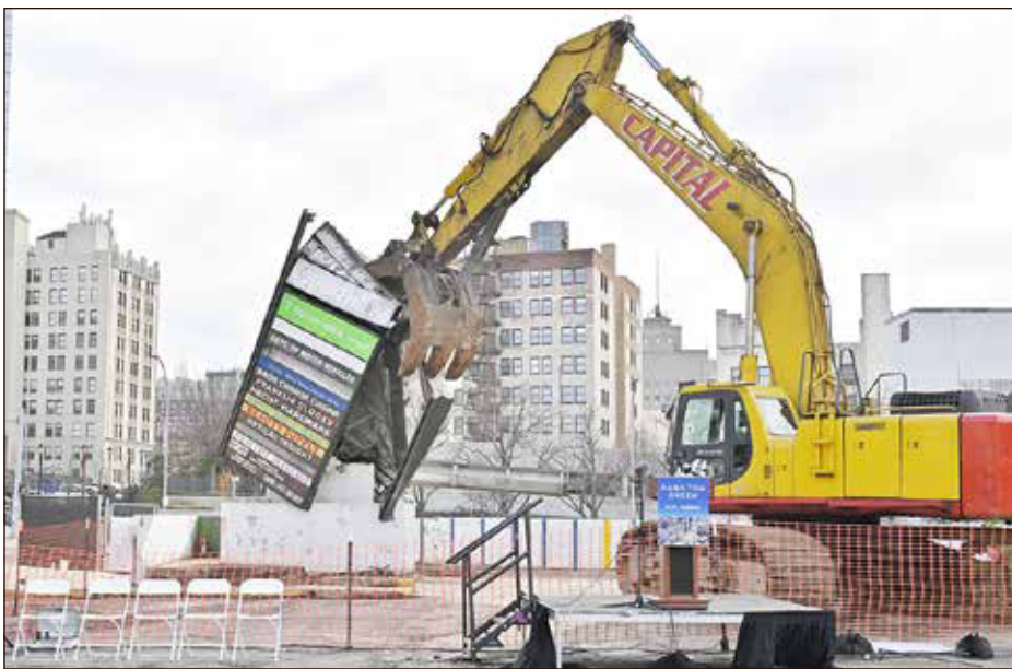
The demolition of the White Plains Mall sign.
