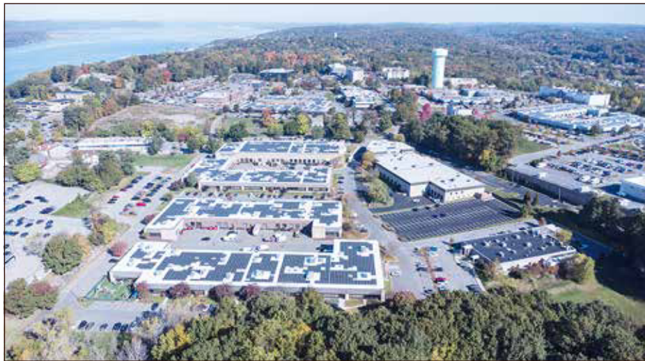
Robert Martin has installed rooftop solar at its properties in Westchester, including South Westchester Executive Park in Yonkers (pictured above).
