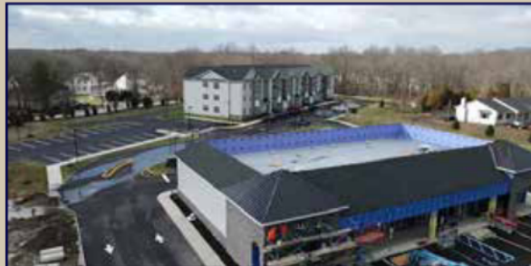
$9.5M 1st - Mixed-use Development Old Bridge, NJ
