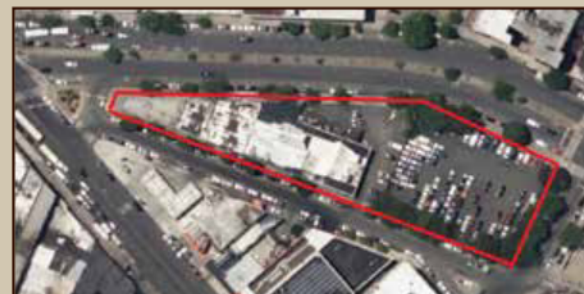
$23.6M 1st - Development Site Bronx, NY
