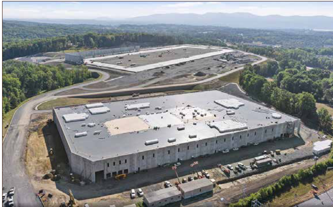
Tesla plans to take occupancy of its Newburgh facility by the end 2023.
