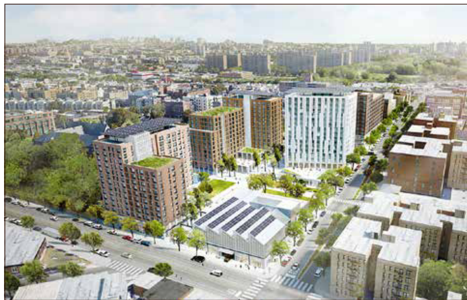
An aerial view of The Peninsula, a 100% affordable mixed-use development in the Hunts Point section of the Bronx. —CREDIT: WXY Studios
