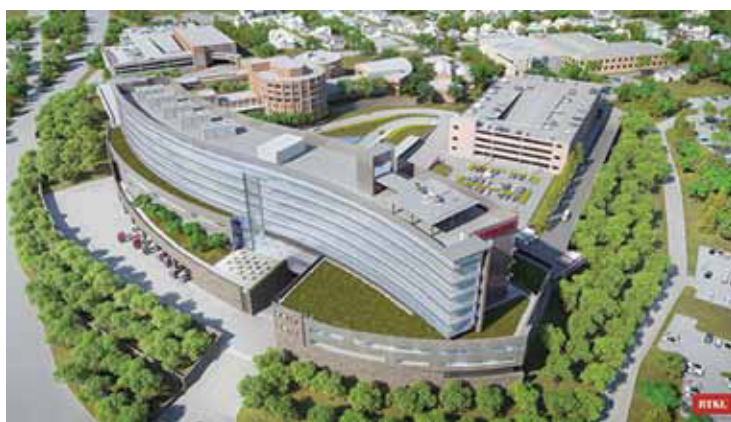
A rendering of the $466-million Vassar Brothers Medical Center Patient Pavilion in Poughkeepsie.
