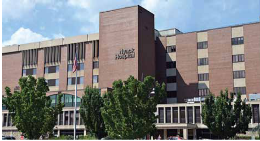
Nyack Hospital is set to commence its ambitious Care Transformation Project that includes the construction of a two-story addition, which will double the size of the existing Emergency Department and add a new Medical Village. The hospital secured CFA funding for its Transitional Care Unit on the fourth floor 4-Maze Nursing Unit.
