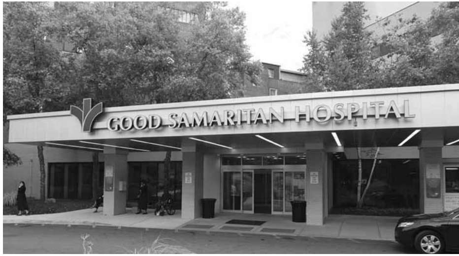
Good Samaritan Hospital in Suffern is part of the Bon Secours Charity Health System.
