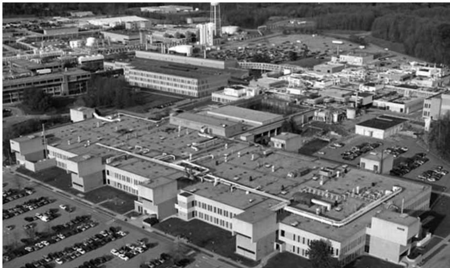
An aerial view of the former IBM East Campus in East Fishkill in Dutchess County.
