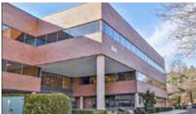
ROCKLAND EXECUTIVE CENTER 100 DUTCH HILL ROAD, ORANGETOWN, NY UP TO 2,500SF FOR LEASE | STARTING AT $23/SF NNN
