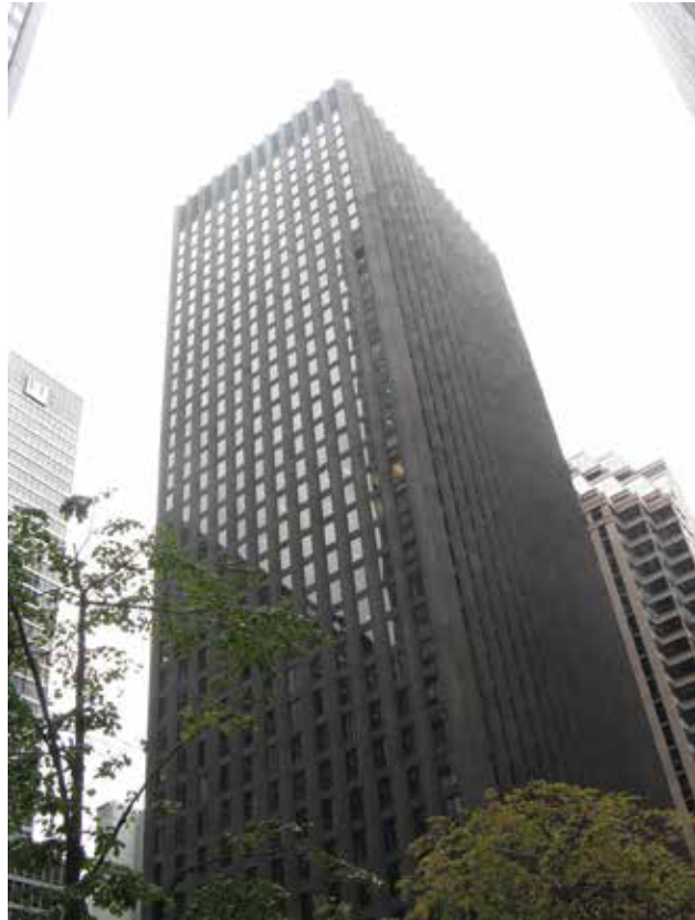
The CBS Building in New York City at 51 W. 52nd St.
