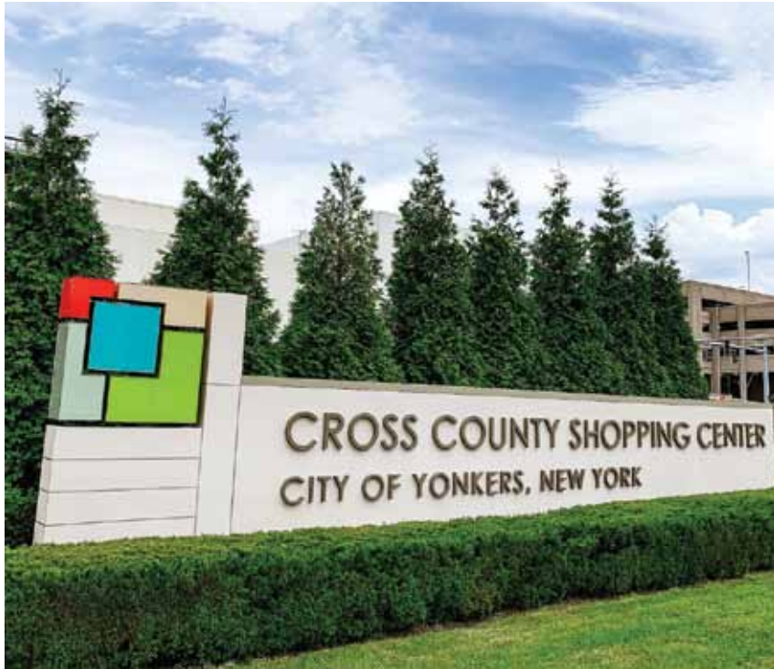
The ownership of the Cross County Shopping Center is now tackling the redevelopment of a former Sears store.
