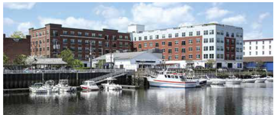
The Mariner is a 100-unit multifamily property located along Port Chester's waterfront.
