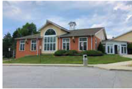
SINGLE TENANT INCOME PROPERTY WITH UPSIDE IN STRONG LOCATION FOR SALE | 48 Route 6 | Yorktown Heights Listed by Steven Salomone | $2,990,000
