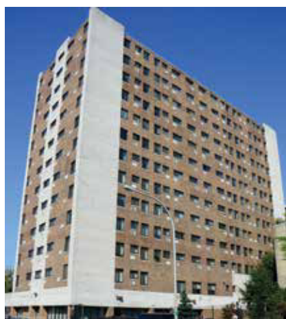
The Hudson Valley Property Group is acquiring the 12-story Jackson Terrace Apartments in Yonkers.
