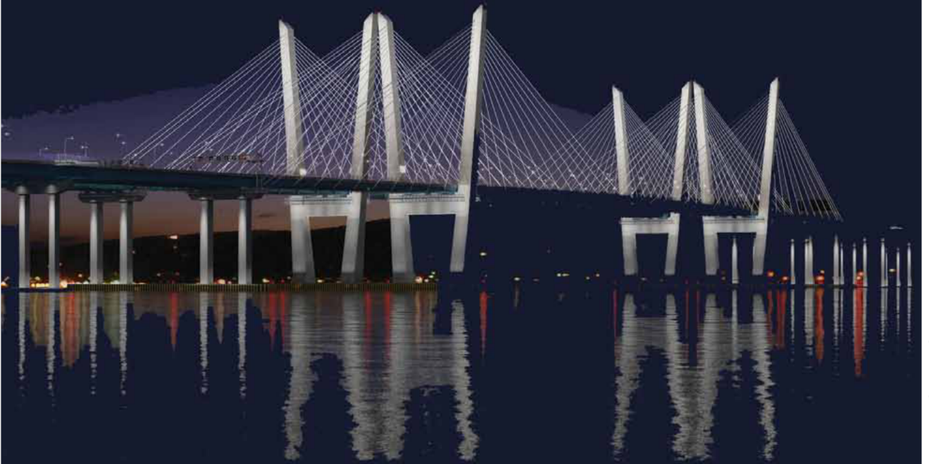
Photo Credit: New York State Thruway Authority
