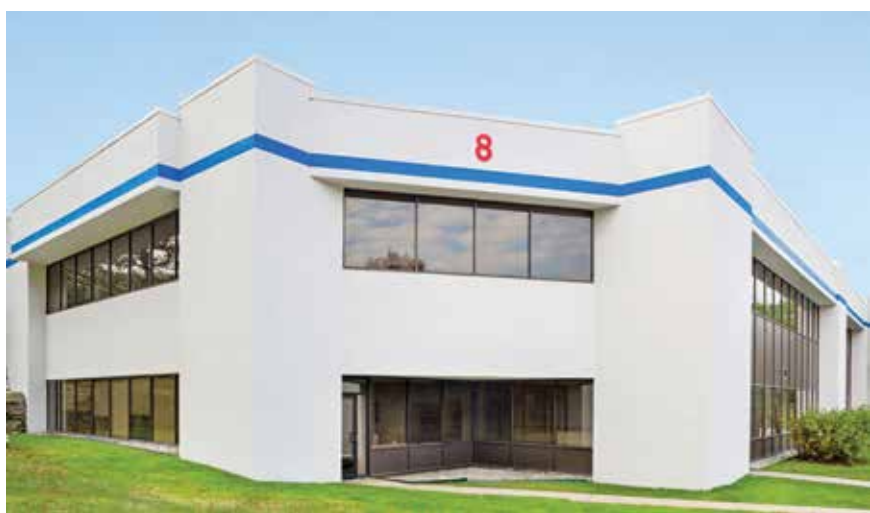
With its new lease deal, PTI now occupies approximately 28,000 square feet of space at Robert Martin Co's 8 Skyline Drive in Elmsford.
