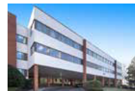
LOCKWOOD MEDICAL CAMPUS NEW ROCHELLE NY 1,000 TO 26,000 SF AVAILABLE $26.00/PSF + ELECTRIC
