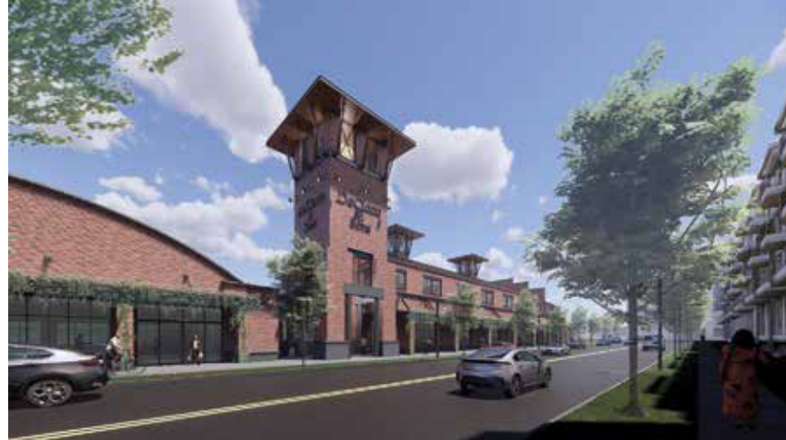
A rendering of the 30,000-square-foot DeCicco & Sons market to be built at the Edge-on-Hudson development in Sleepy Hollow.
