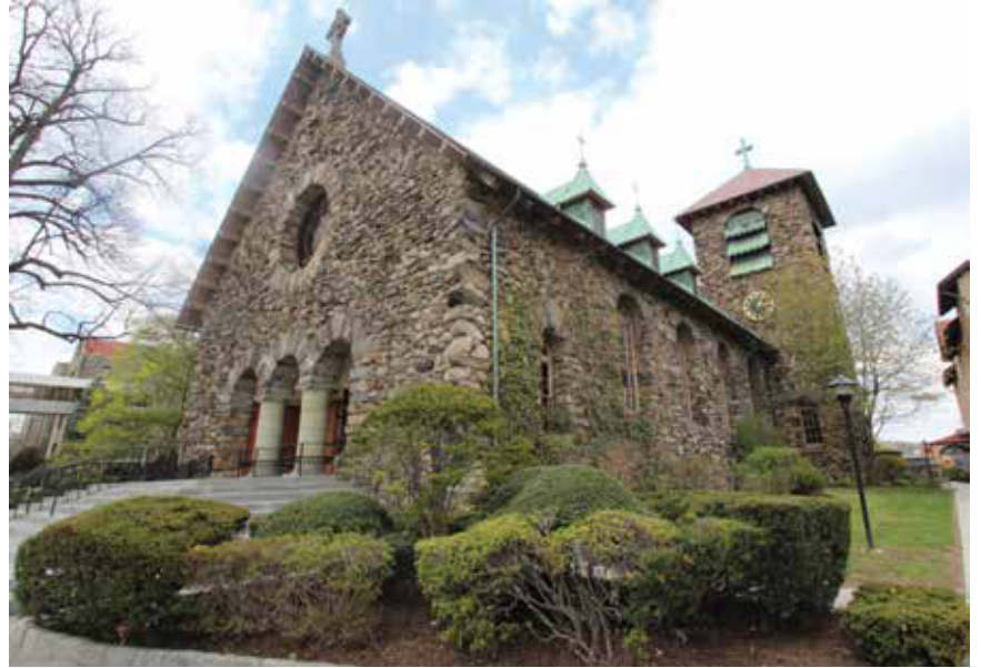
The plan calls for the preservation of the Chapel of the Sisters of Divine Compassion at the former Our Lady of Good Counsel property at 52 North Broadway in White Plains.
