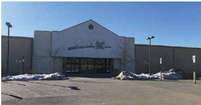
The former K-Mart store in Yorktown Heights could be razed to create a new residential development.
