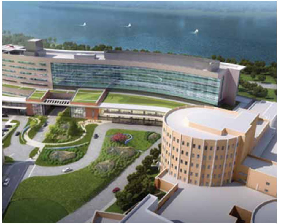
Vassar Brothers Medical Center is seeking $18.4 million in CFA funding in connection with its campus expansion in Poughkeepsie. The total project is reportedly valued at $466 million. Construction began on the project in September.
