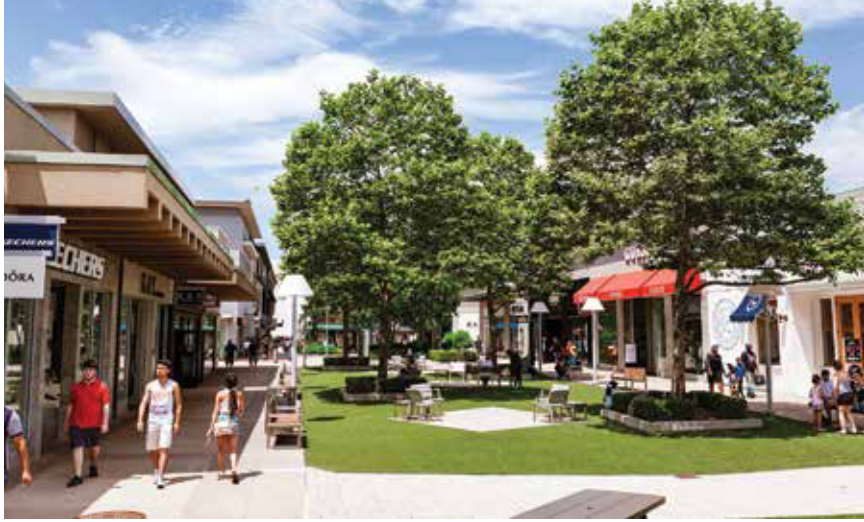
The ownership of the Cross County Center is engaged in a multi-phased plan to reimagine the nation's first open-air shopping center.
