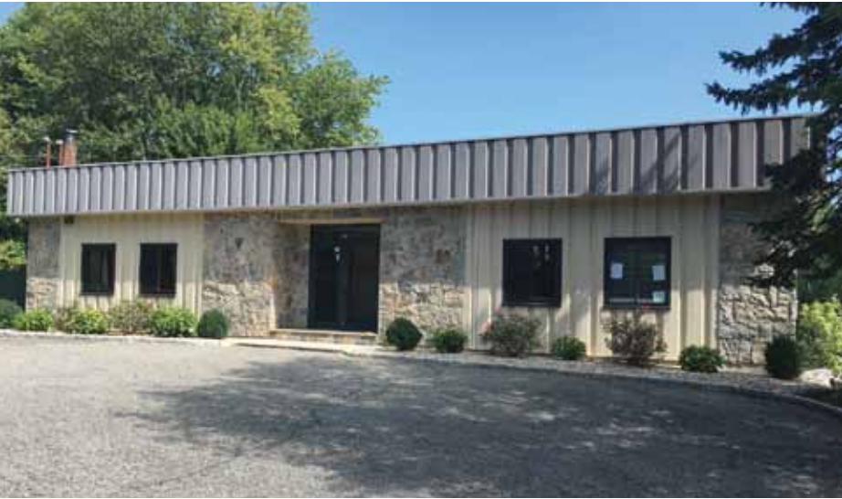
The Laborers Local No. 60 Training & Education Center building in Brewster.
