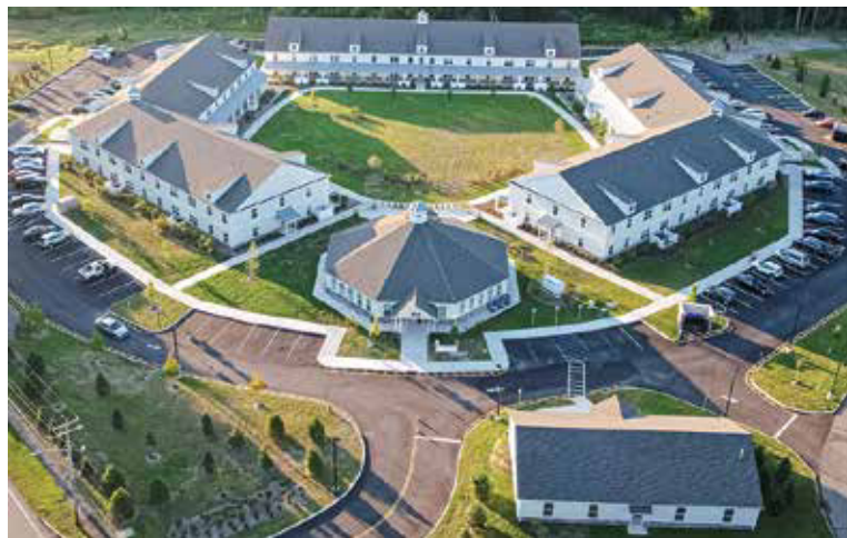
Vincent's Village totals 93 units of affordable senior housing in Nanuet.
