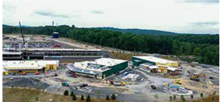
The LEGOLAND construction site in Goshen.
