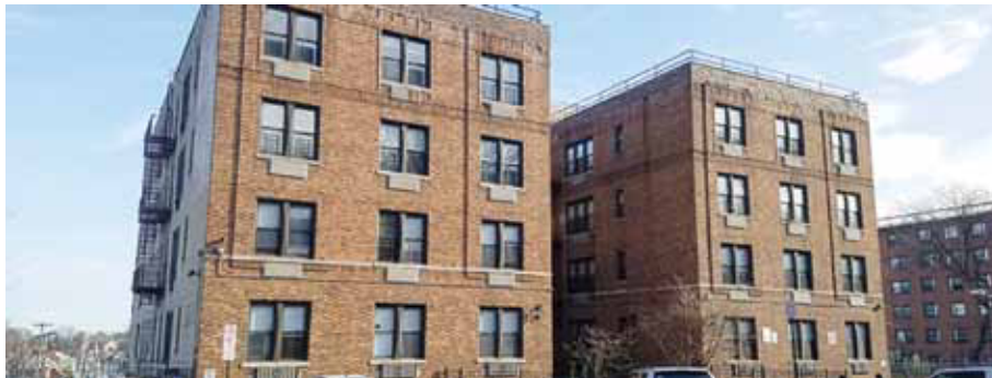
21 Fountain Place formerly served as student housing for Monroe College in New Rochelle.
