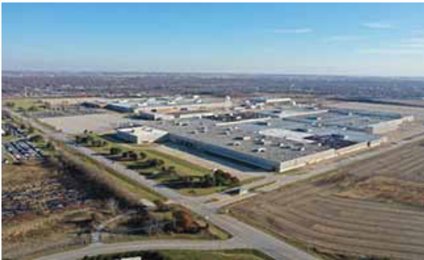
The four-million-square-foot Caterpillar campus in Montgomery, IL.
