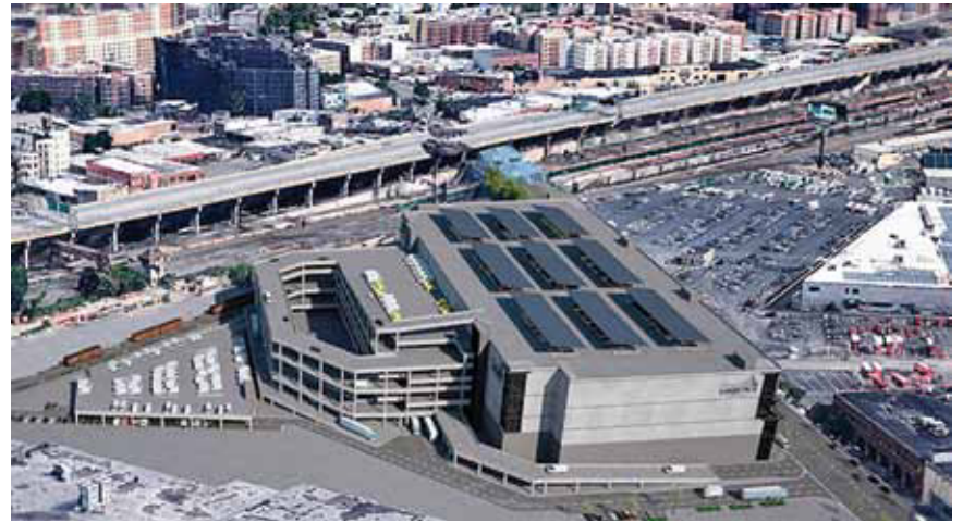
A rendering of the 1.24-million-square-foot Bronx Logistics Center in the South Bronx.
