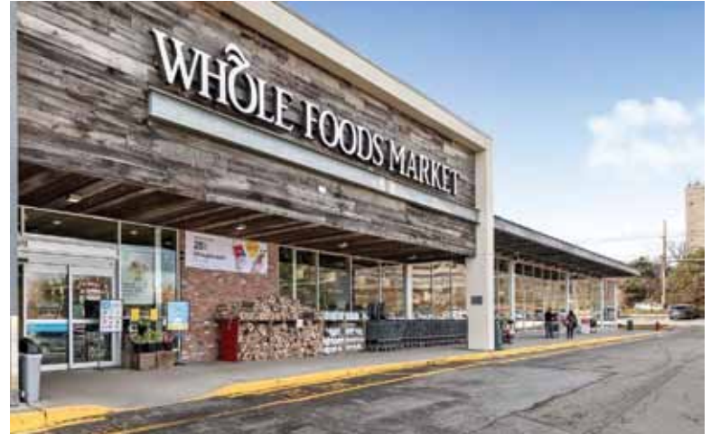
Whole Foods is an anchor at the Port Chester Shopping Center.
