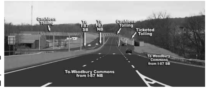
A rendering of some of the planned improvements to the Harriman toll interchange adjacent to Exit 131 of Route 17.
