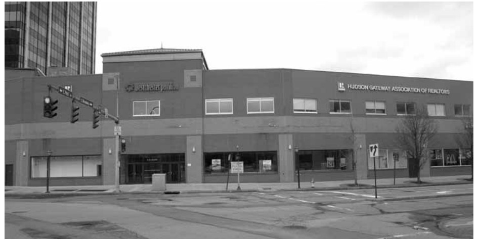
The Westchester Pavilion mall in White Plains will be demolished to make way for a mixed-use development featuring rental apartments and retail space. FILE PHOTO
