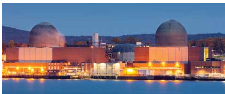
The two operating nuclear reactors at the Indian Point Energy Center will cease operation by 2021.
