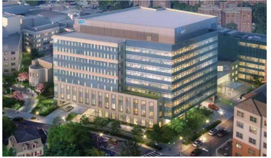
A rendering of the new White Plains Hospital outpatient center for advanced medicine and surgery, which is now under construction.
