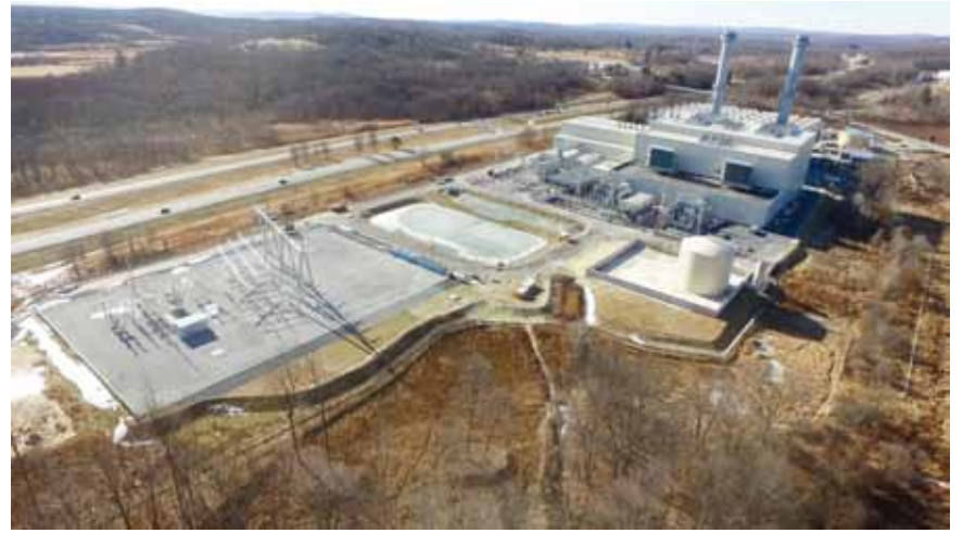
An aerial view of the CPV Valley Energy Center in Wawayanda.
