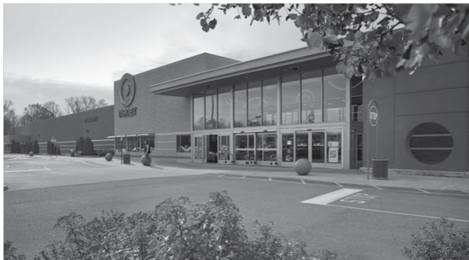
The Morris Companies' 348,312-square-foot portfolio in Yonkers includes Stew Leonard's, Costco and Home Depot and is fully leased. The photo above is a Target store in the Morris Companies' portfolio in Heritage Square, South Brunswick, NJ.
