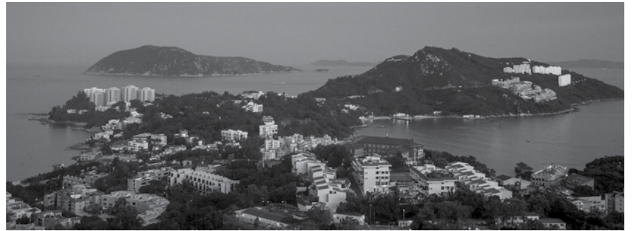
An aerial photo of the Stanley Hilltop property in Hong Kong.
